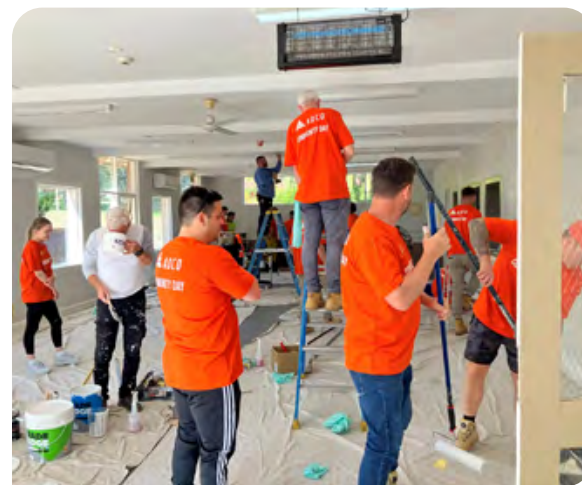
>> The ADCO team working on the dining room space at Harry Hunter Recovery Centre in Perth.
