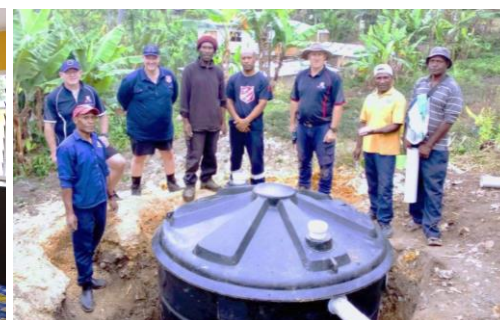
Installing a septic tank
